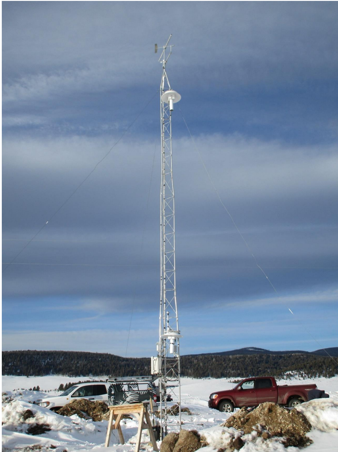
Figure 3. Photo of Meteorological Tower at New Location
